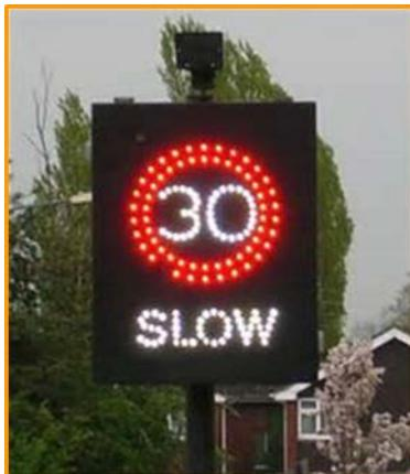
The Moveable Vehicle Activated Sign (MVAS) initiative is a locally managed scheme where rechargeable vehicle activated signs can be purchased by the Parish/Town Council and moved around the village to pre-agreed locations, co-fixed onto existing posts or onto a movable post secured by a ground screw.
